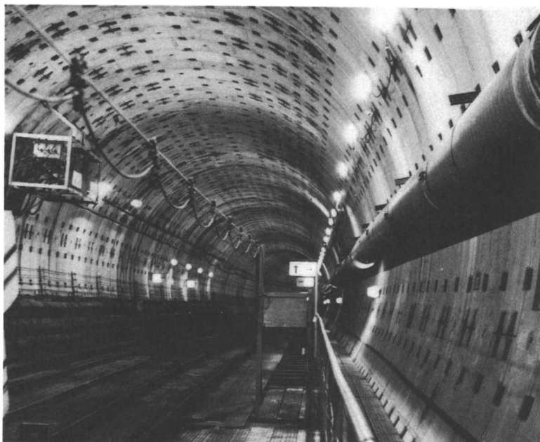
Fig. 6 A tunnel constructed with segments. (Reproduced with permission from ref. 3. Copyright 1991 T. Konno)
